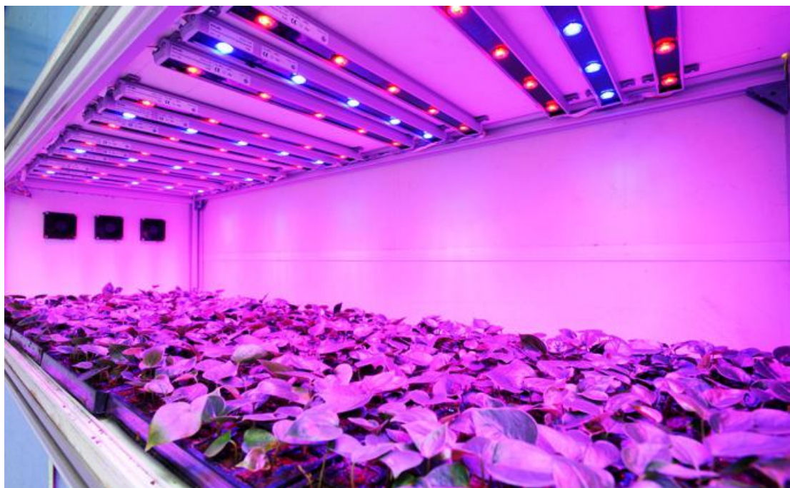
Red and Blue LEDs being used together for plant growth. Image courtesy: www.uponics.com
