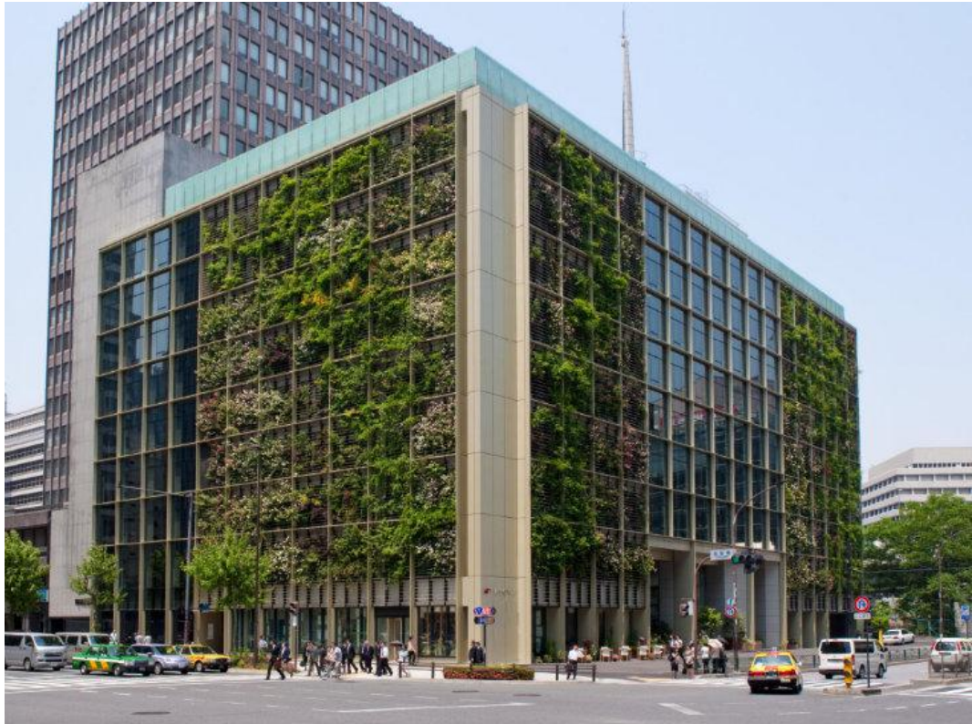
Facade of the Pasona HQ in Tokyo. Image courtesy: www.konodesigns.com
